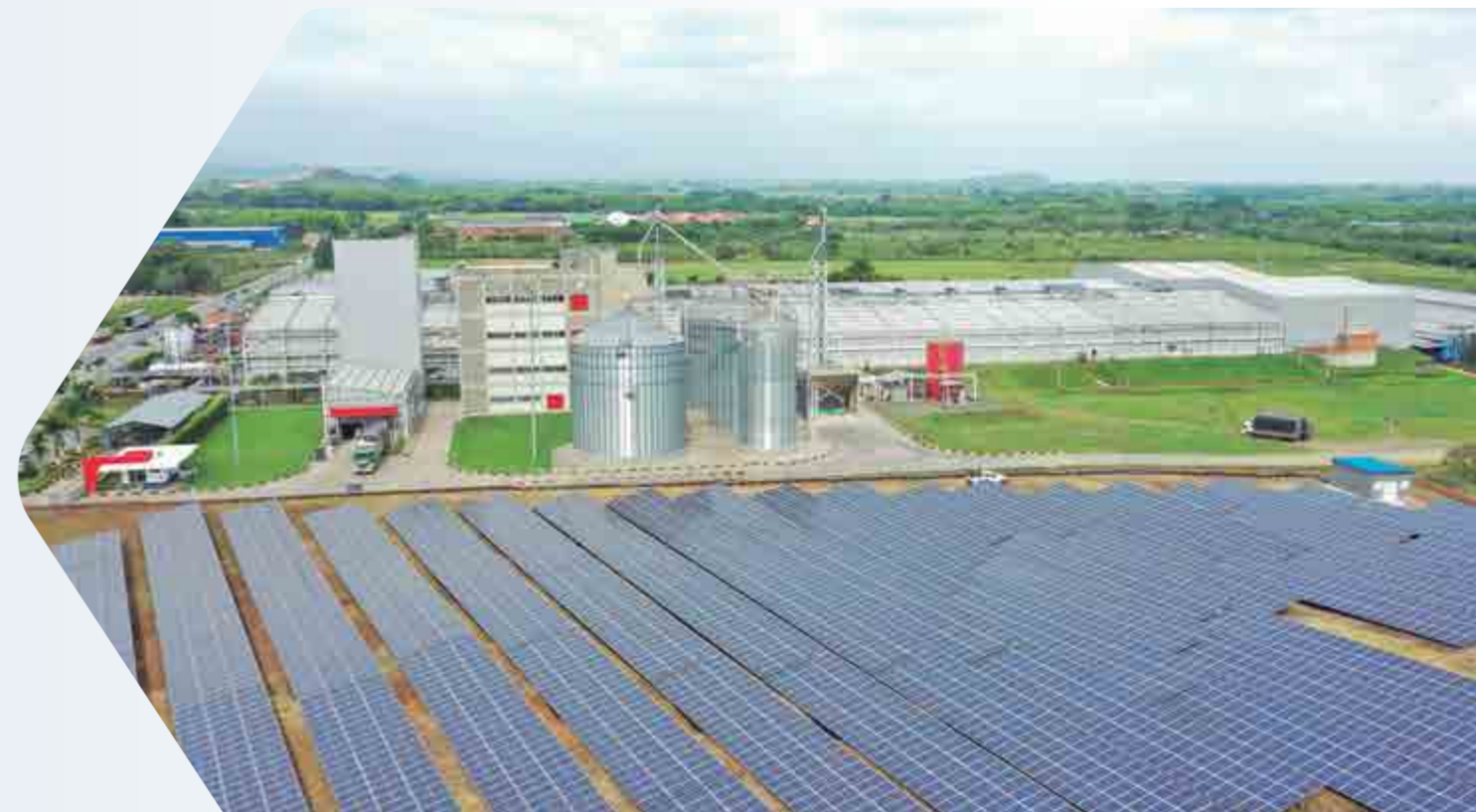
Solar Farm, Cookies and Crackers Plant, Santander de Quilichao.
